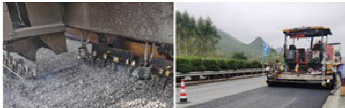
Guilin Subsidiary Applying Hot In-place Recycling
