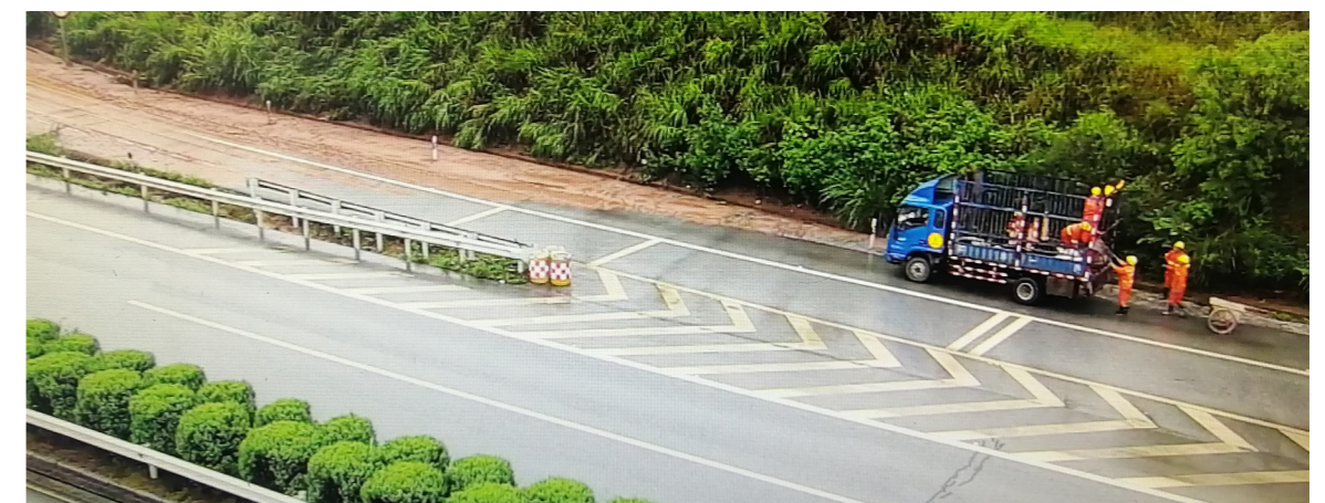
Flood Control On-site Operations by Guilin Subsidiary
