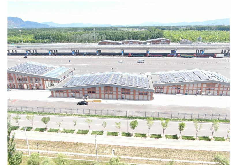
Rooftop Solar Panels of Beijing-Chongli Expressway Banquan Service Area
