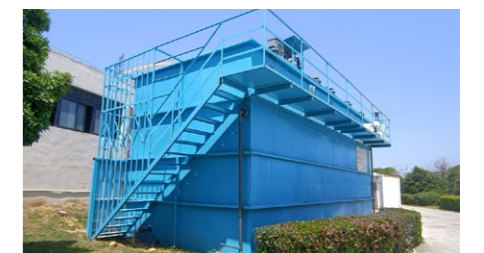
Sewage treatment project of Ningbo-Taizhou-Wenzhou Expressway
