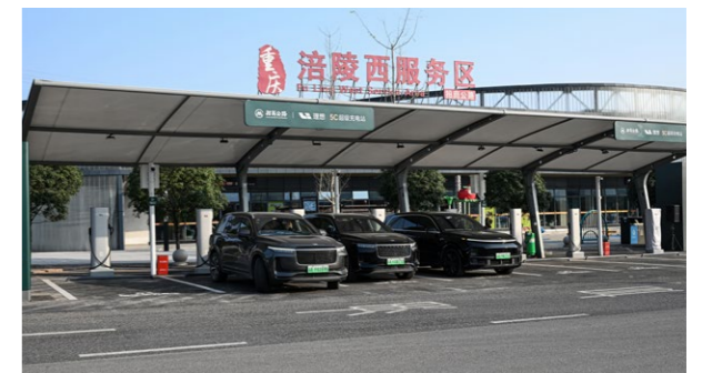
Fuling West supercharging station
