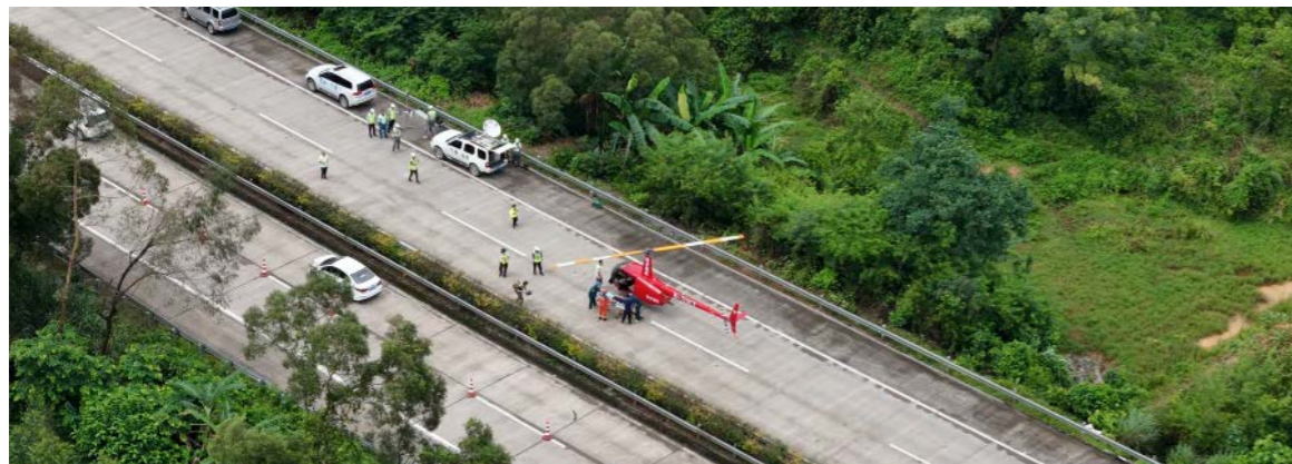
On-site emergency drill addressing rainfall-induced slope collapse incident
