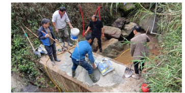
Water saving construction at the Yanglushan tunnel of Chongqing subsidiary
