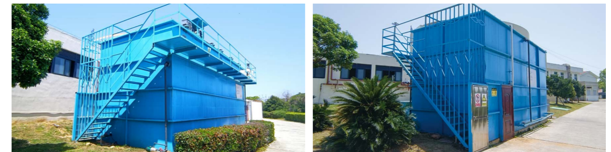
The "reclaimed water" sewage treatment system of Ningbo-Taizhou-Wenzhou Expressway
