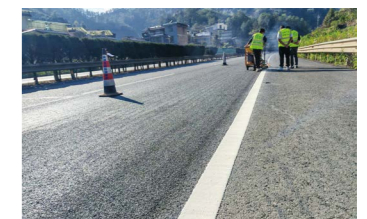
The subsidiaries' on-site application of restoring existing road marking technology
