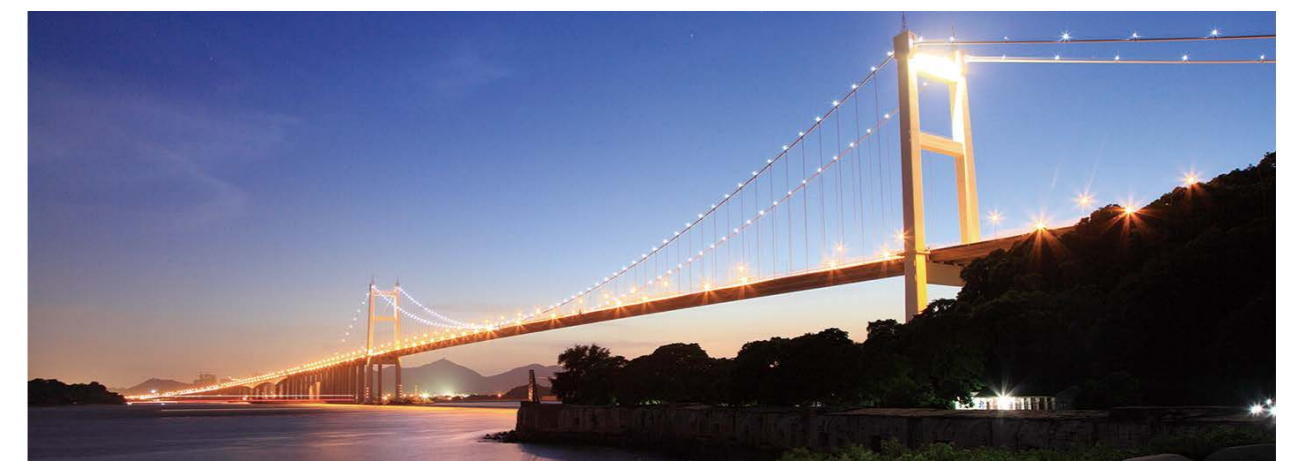
Humen Bridge Main Cable
