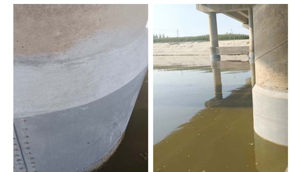
High-Strength Steel Wire and Fiberglass Sleeve Reinforcement System of CMCR
