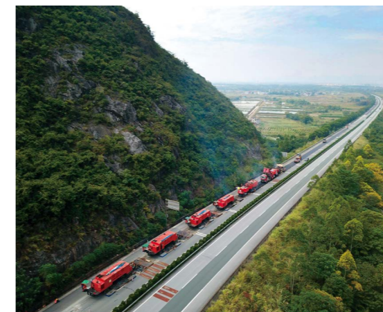
The subsidiaries' on-site hot in-place construction
