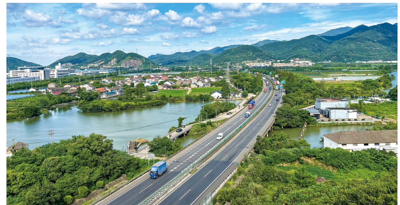
The first section of the Ningbo-Taizhou-Wenzhou Expressway in Ningbo
