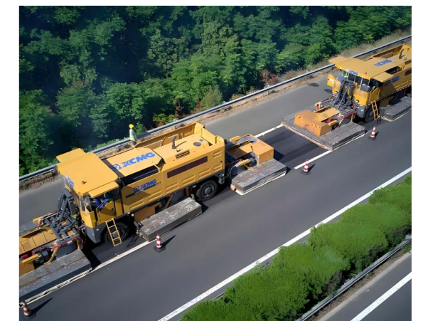
The subsidiaries' on-site hot in-place construction
